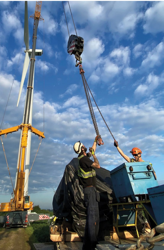
LEFT The team prepares for a gear box replacement at Erie Shores Wind Farm. RIGHT Gearing up with PPE for electrical work.
