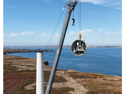
The nacelle is removed from a tower being decommissioned at our Glace Bay wind facility (Nova Scotia).
